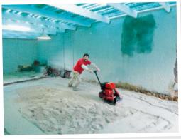
ABOVE LEFT The sunken floor in the dining room was filled in with rubble. LEFT Thabo compacted the floor of the new living area and braai room which was built on outside the dining room.
