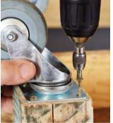
$\bf 6$  Place the cupboard upside down on the top assembly and position it so that the top has an equidistant lip all round. Attach with the 8mm x 50mm screws. Attach a castor to the bottom of each leg.
