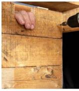
**3** Screw the five 350mm planks to the inside of the legs on the 'left' of the cupboard – make sure the ends of the plank are flush with the 'front' leg edge. Cut out a small section of the top plank for the gas pipe.
